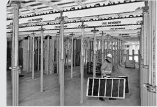
Slab Formwork
